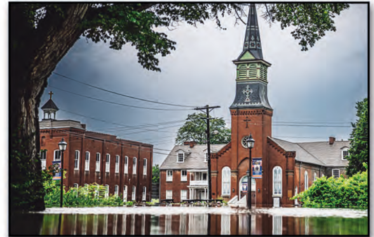
The Devasting Flooding that Occurred in July of 2022 Old St. Ferdinand Shrine was Extensively Damaged The Shrine Welcomes Any Donations and Assistance
