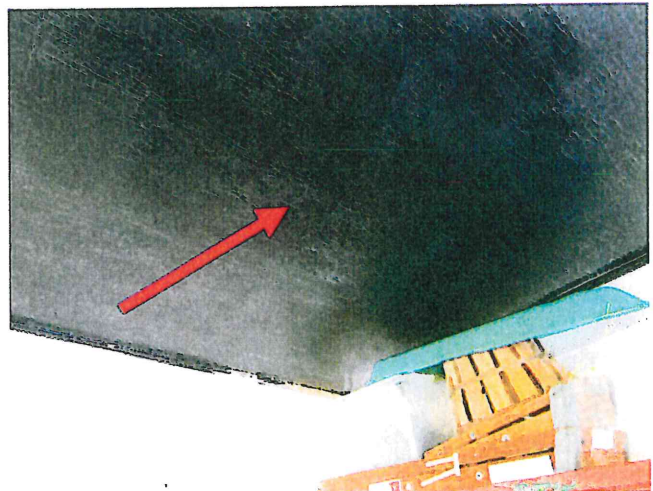
Photo 6: Carport Upper Ceiling
