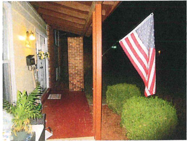
Photo 4: Front Porch Post (Side View)
