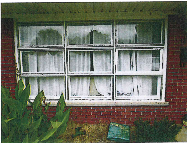
Photo 5: Window System (#1-3, #4-6, and #7-9)
