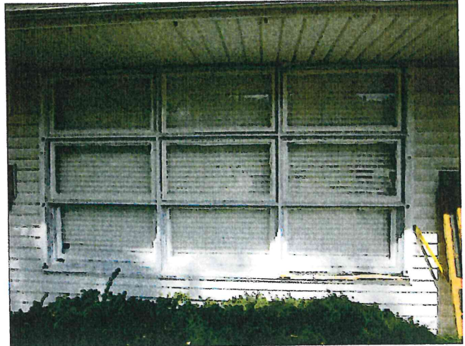
Photo 2: Window System (#1-3, #17-19, and #20-22)
