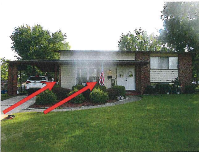
Photo 3: Front Porch Posts #1-4
