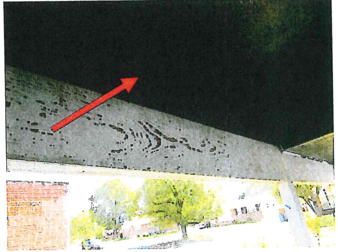
Photo 2: Carport Upper Wall (D-wall)
